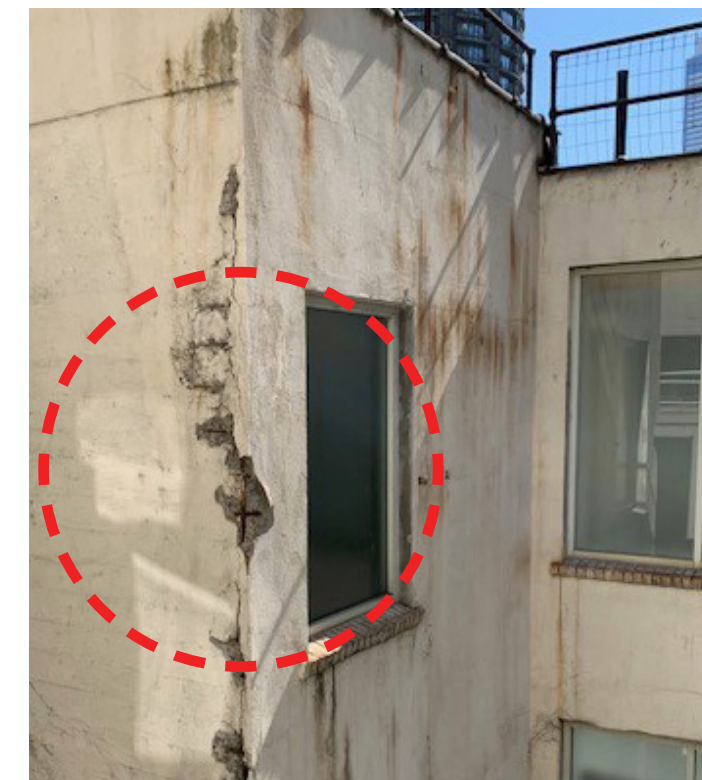
RUSTED/EXPOSED STEEL
