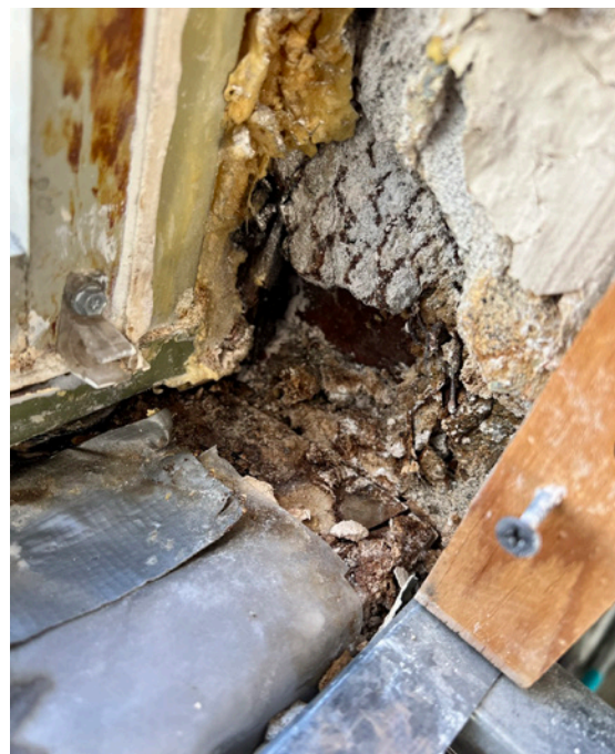
GRIFFIN & SHERIDAN STRUCTURAL CONDITIONS
