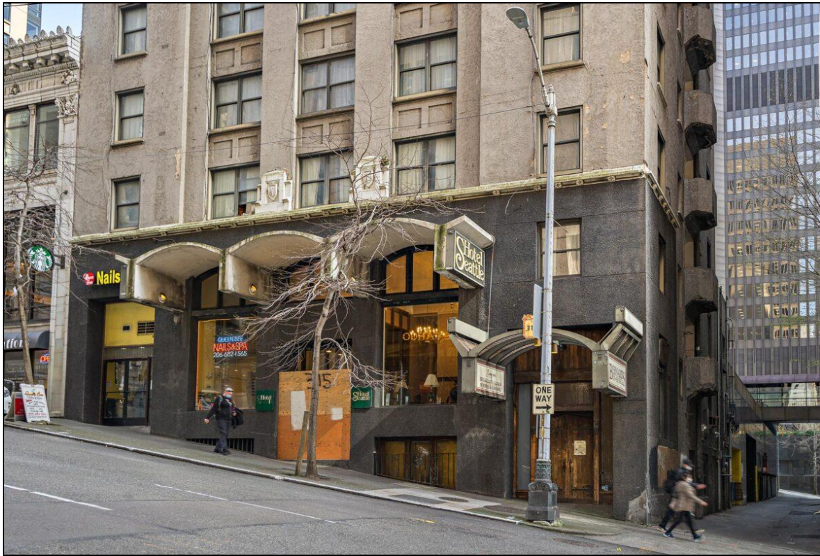
Figure 51. Above, the lower level, north façade with its three thin shell canopies. (Kidder Matthews photo, 2020) Figures 52 & 53. Below left, detail view of the lower steel canopy. Right, the base and sidewalk.
