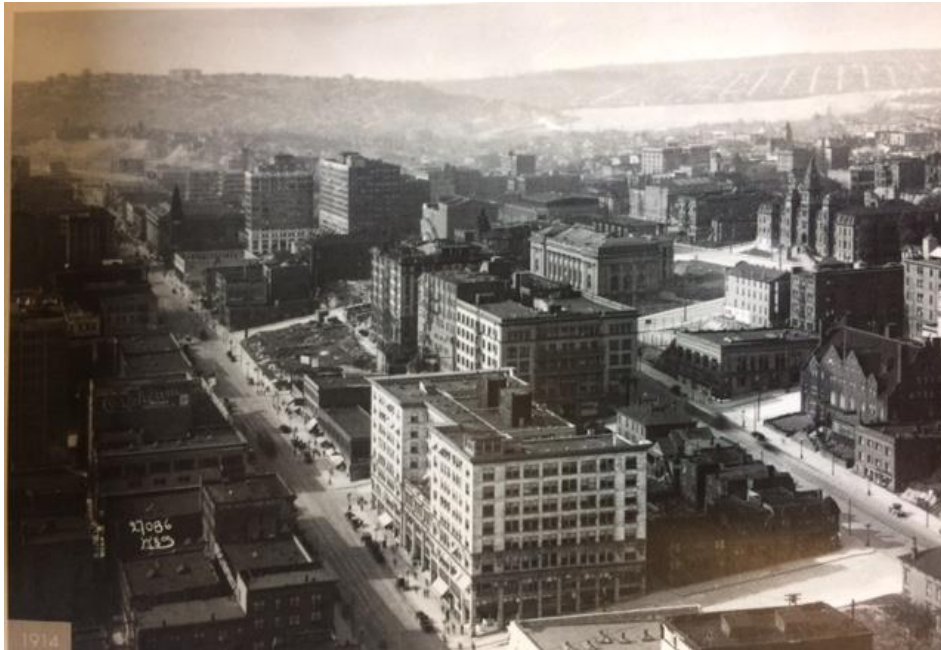
Figure 7. Above, looking north along 3 rd Avenue north of James Street in 1914. (SPL, spl_shp7383).
