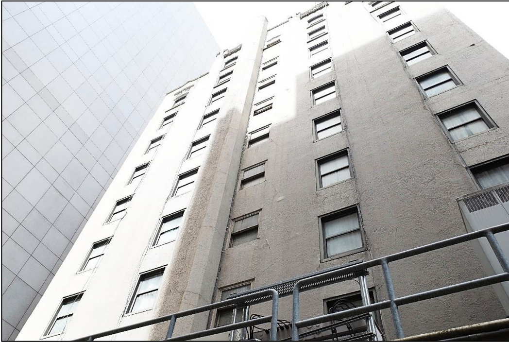
Figure 49. Above, Looking upward at the south façade.
