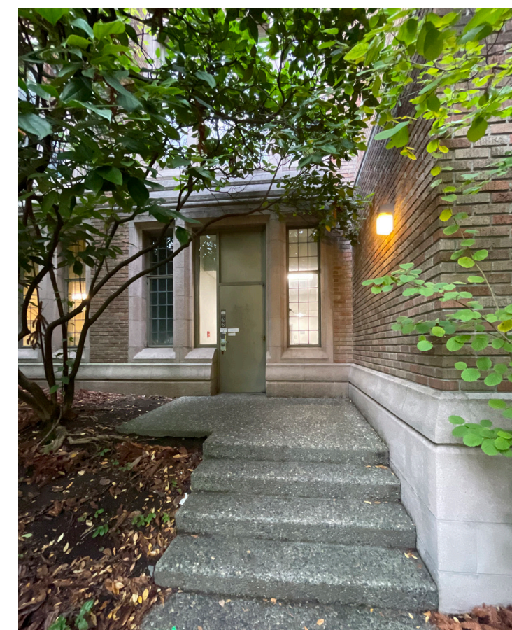
Southwest and southeast entries and stairs added in 1971 after removal of the central entry doors and arcade. Entries currently lack accessibility or strong visual connection.
