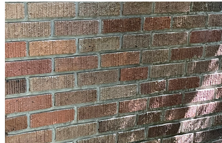
Existing brick detail.
