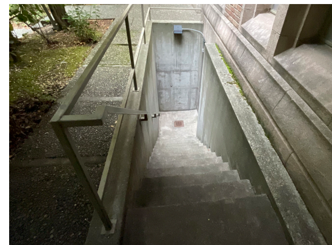
Subterranean mechanical room access stair added in 1971
