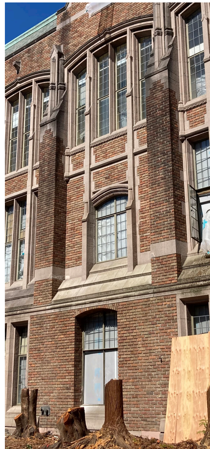
1971 masonry infill and replacement windows at historic south entry
