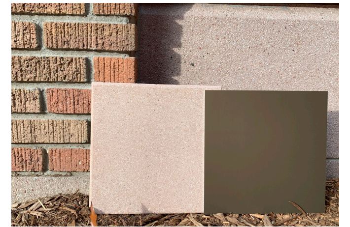
Proposed control sample for M-1 adjacent to proposed C-1, cast stone, and existing historic brick and cast stone.
