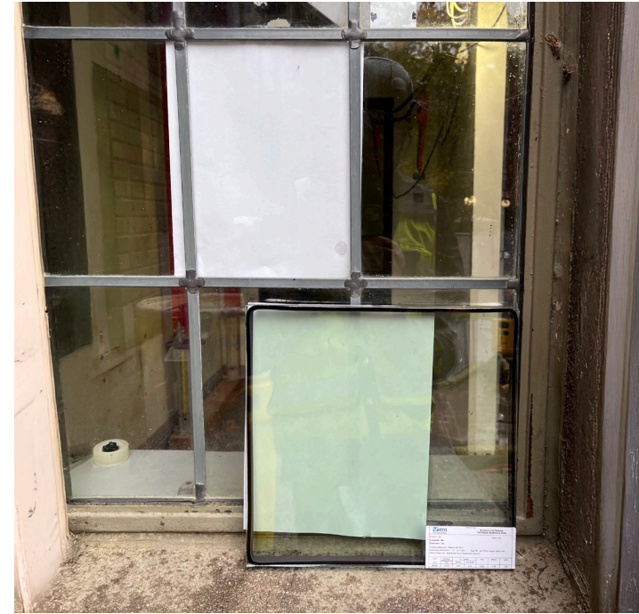
Proposed insulated glazing adjacent to existing historic glazing
