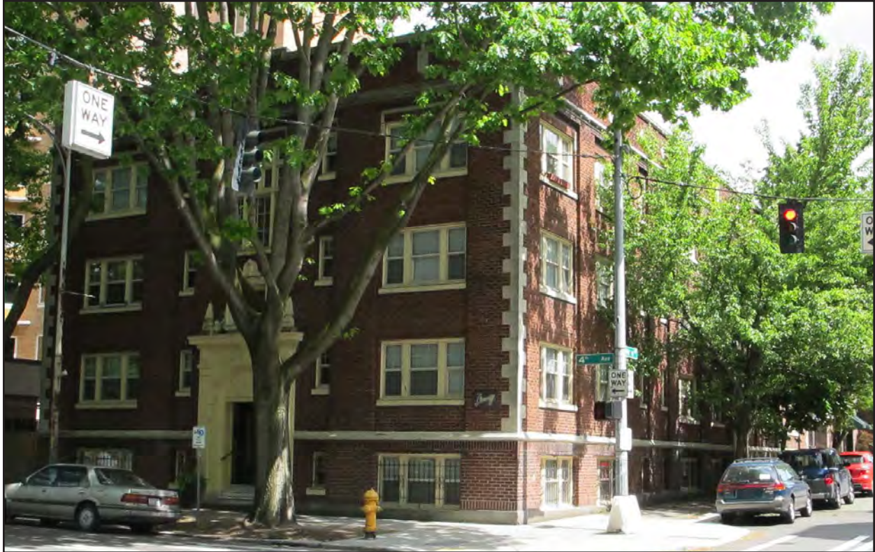
Figure 43 • Stone Cliff Apartments (2602 Fourth Avenue, 1923)
