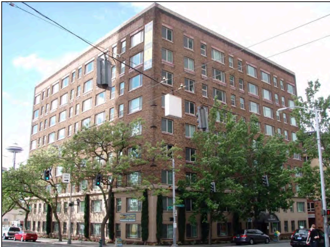
Figure 44 • Cornelius Apartments (306 Blanchard Street, 1925)
