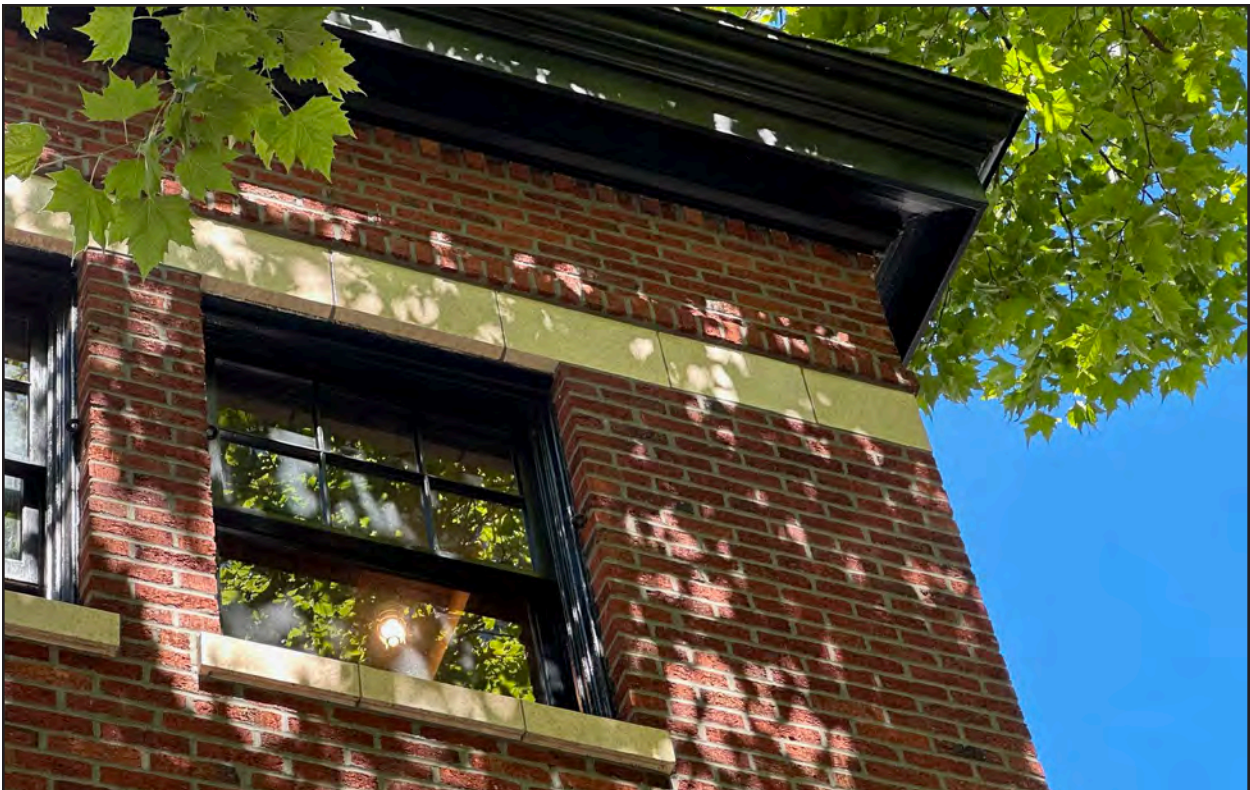
Figure 9 • 2132 Fifth Avenue, western façade, roof detail
