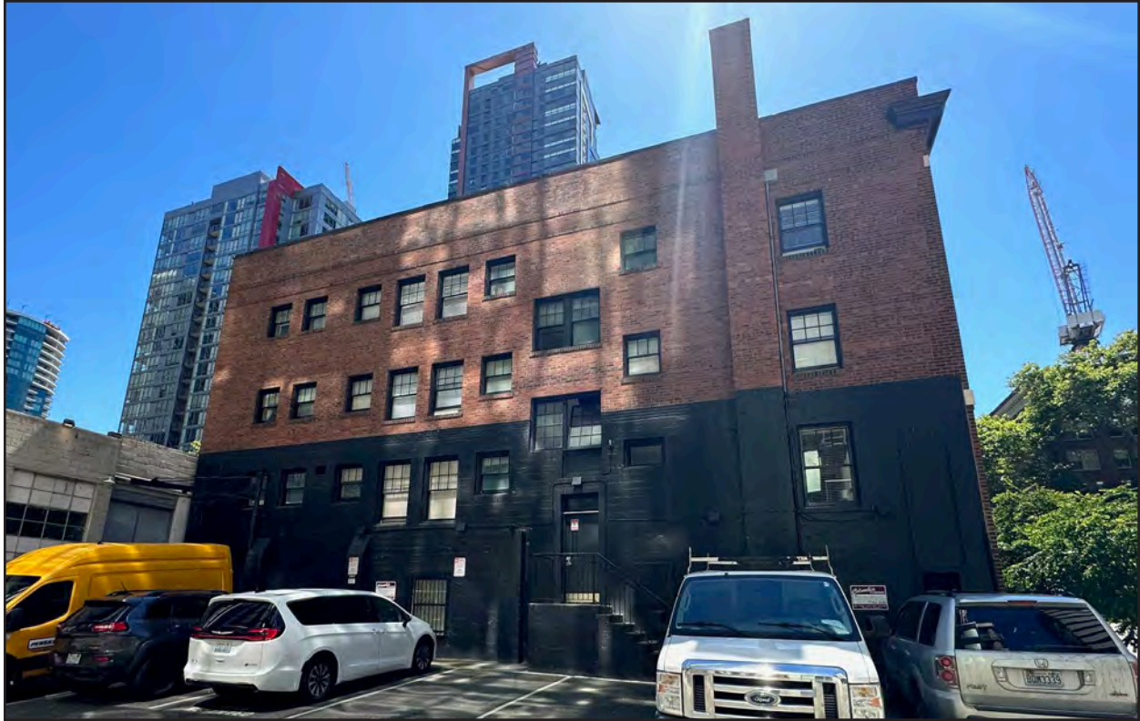
Figure 16 • 2132 Fifth Avenue, eastern façade facing alley
