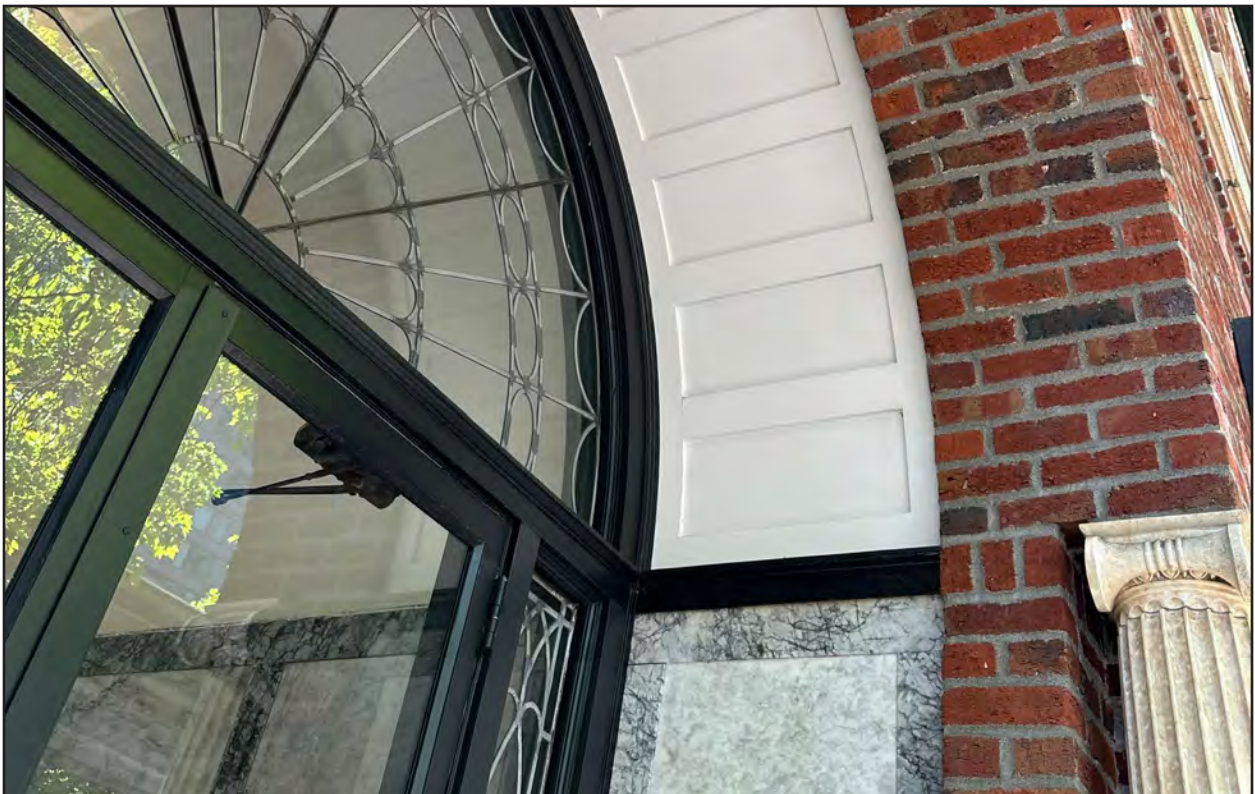
Figure 11 • 2132 Fifth Avenue, western façade, main entrance detail
