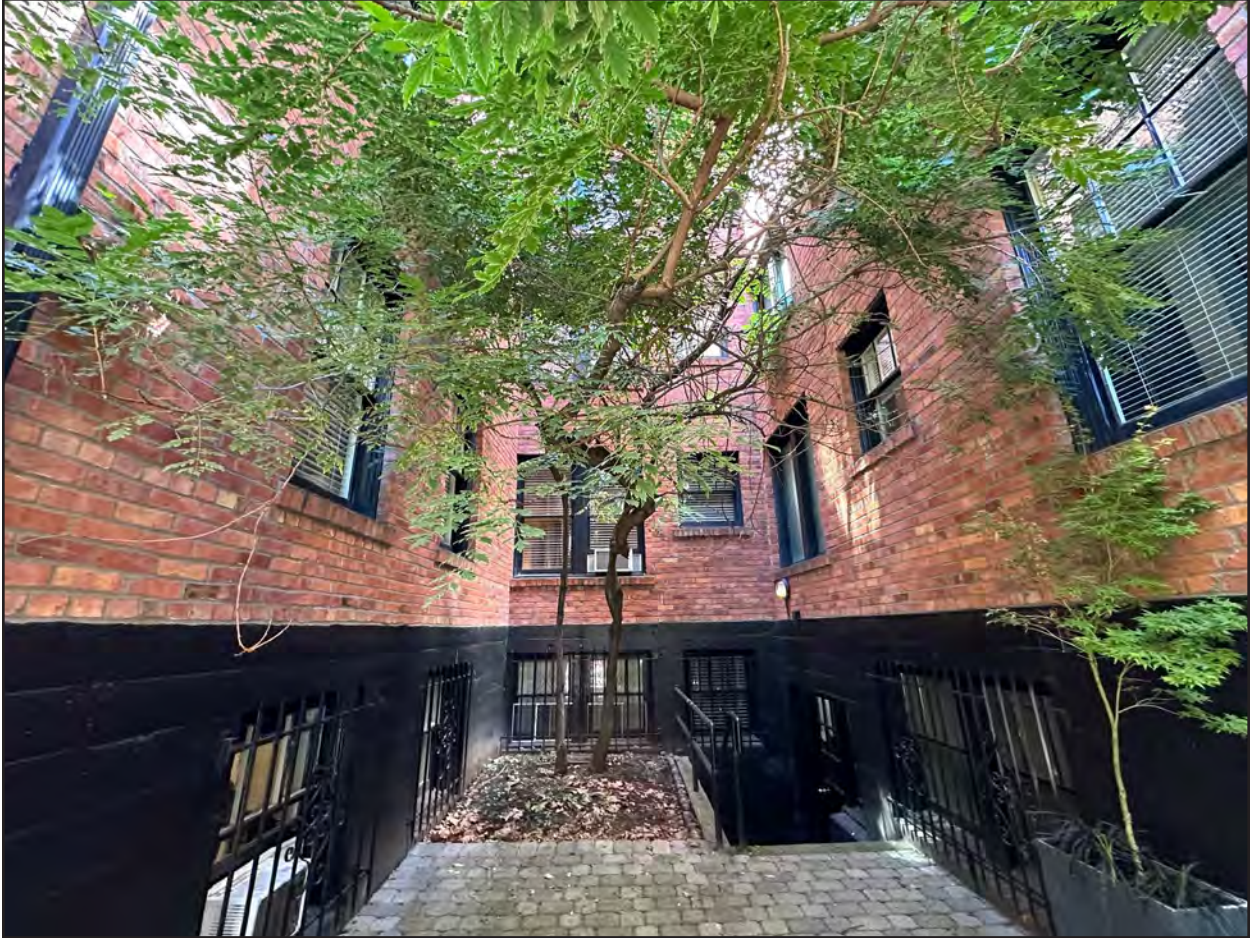
Figure 15 • 2132 Fifth Avenue, courtyard facing north
