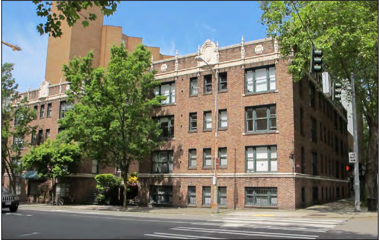
Figure 45 • Davenport Apartments (420 Vine Street, 1925)
