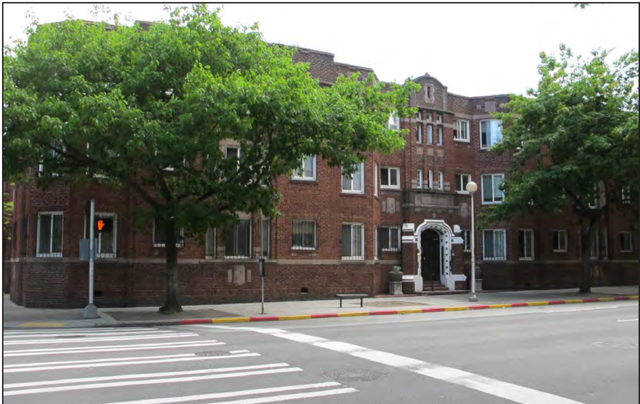
Figure 42 • Charlesgate Apartments (2230 Second Avenue, 1922)
