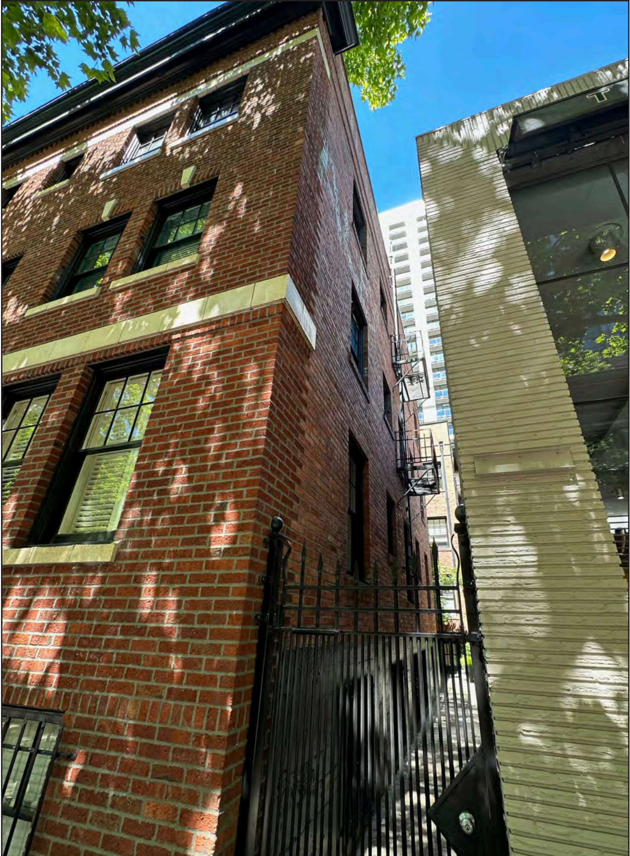
Figure 14 • 2132 Fifth Avenue, southern façade
