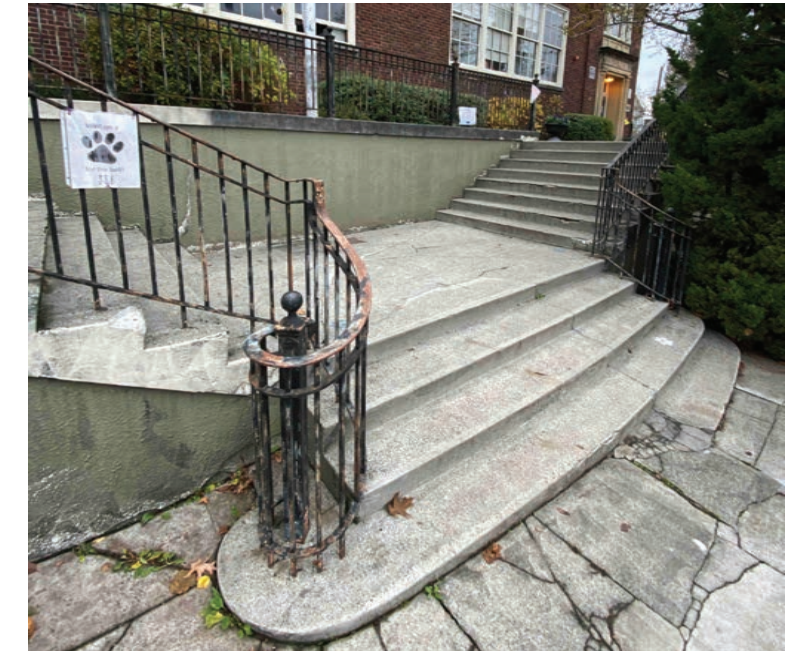
View of existing historic railing at east facade entry
