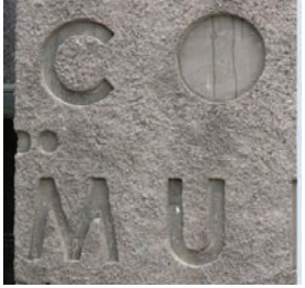
Stamped Concrete Lettering Color: Acid Stained Concrete in dark grey Type Face: Ariel Height: 10" Depth: 1" depression in wall
