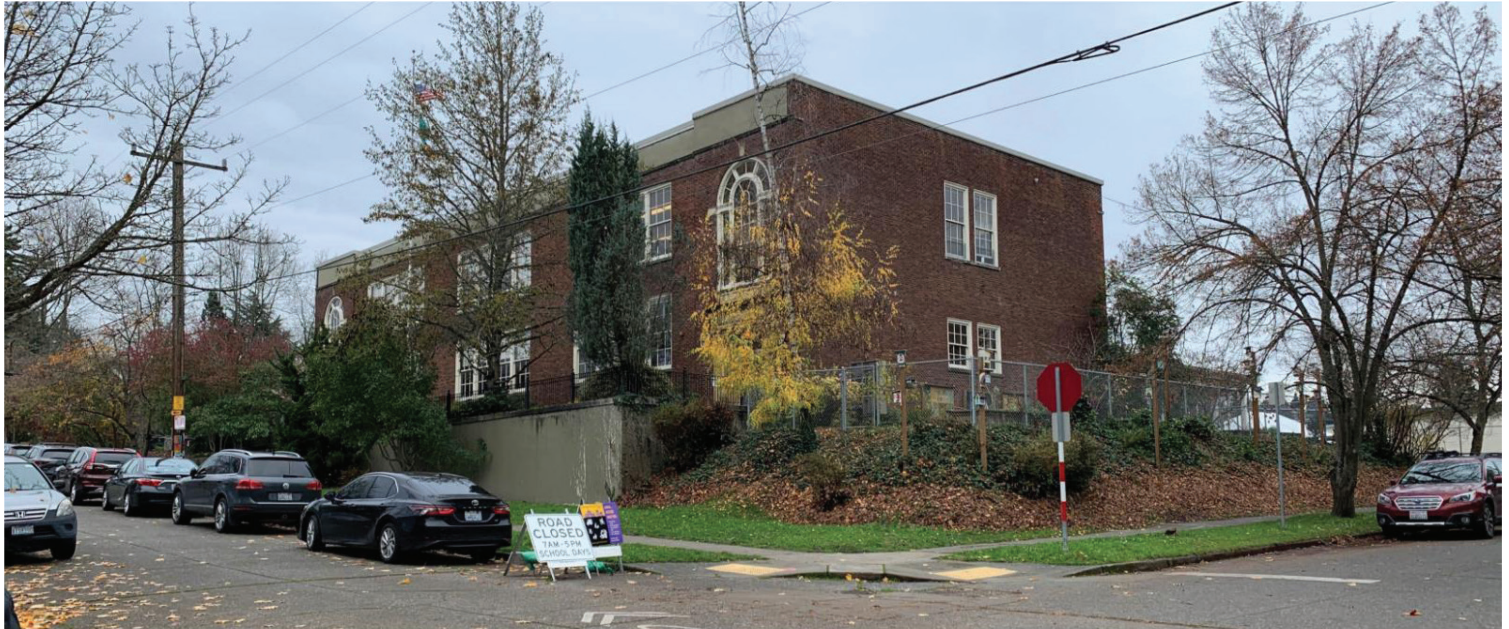
NE View - Corner of 22nd Ave. E and E Calhoun St.
