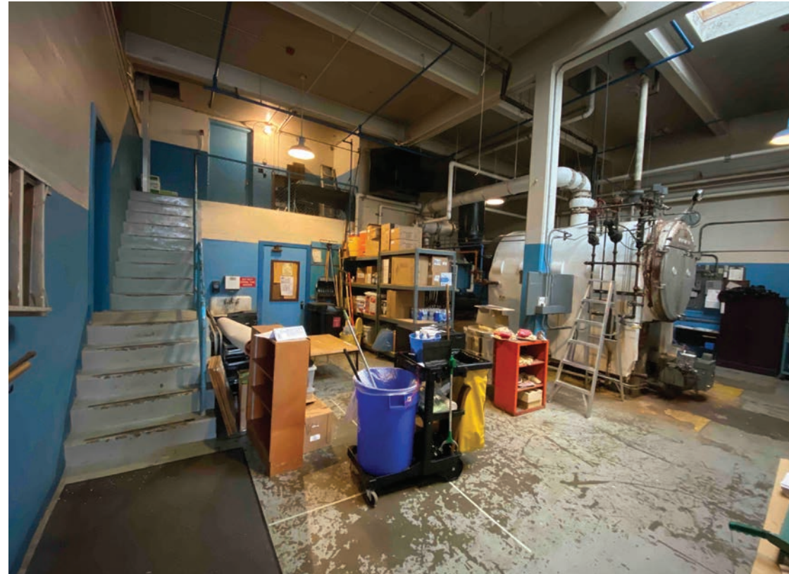
2. Interior view of existing boiler room from bottom of stairs
