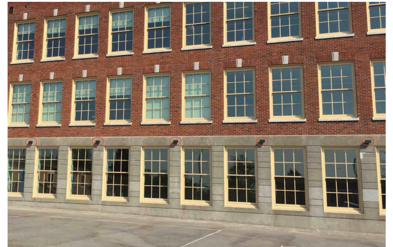
Similar light fixture installation at E.C. Hughes Elementary in Seattle
