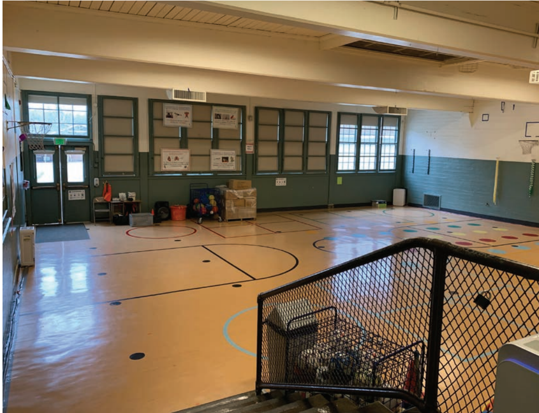
1. Interior view of existing gymnasium from top of stairs
