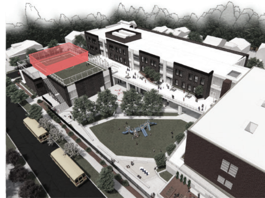
③ PENTHOUSE LOCATED ON GYM ROOFTOP
