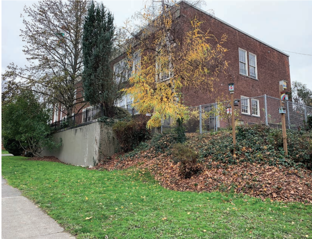
1. View of northeast corner at 22nd Ave E and E Calhoun
