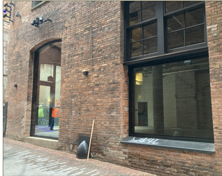
West Facade by Other Building Tenant
