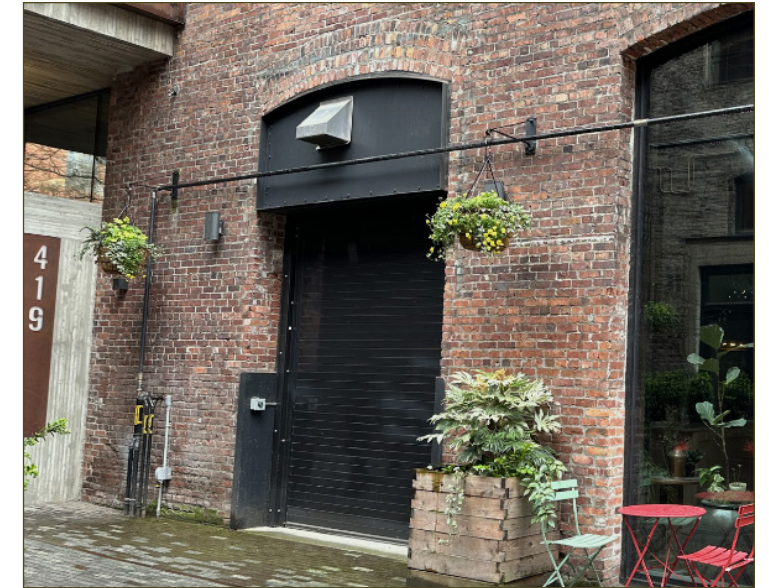
Existing Non-Historic Portion of North Facade
