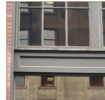
Existing Storefront Black Paint
