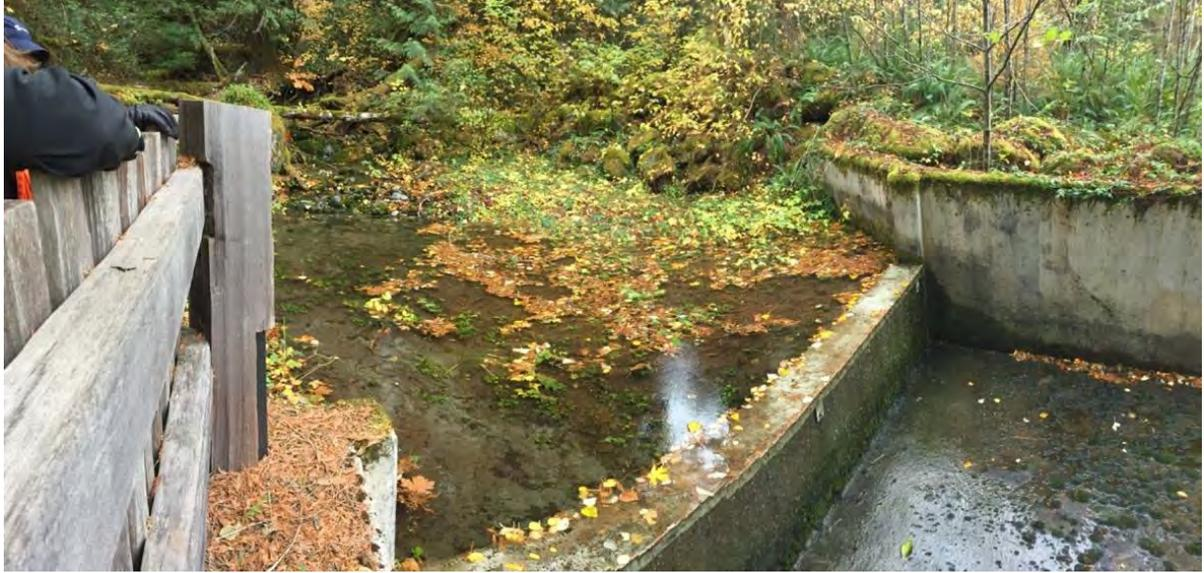
Photograph 9. Surface water features: Fish barrier between powerhouse and Skagit River.
