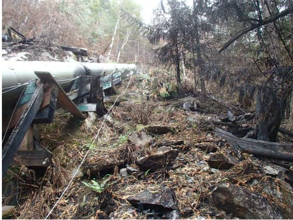
Photograph 1. Two months after the August 2015 Goodell Fire: fire damage at Saddles 46 and 47 prior to the saddle replacement project; view to the south; October 2015.
