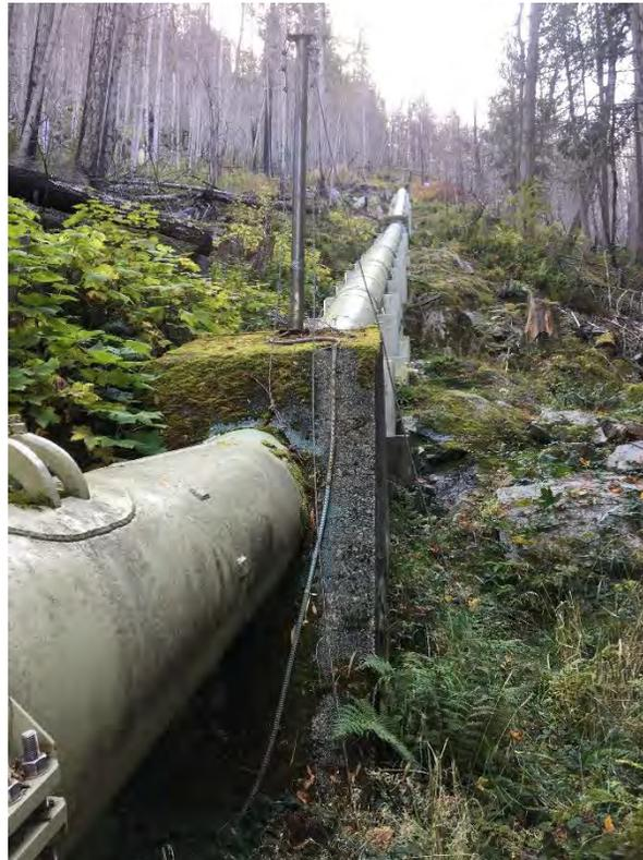
Photograph 10. Thrust Block IV with slight surface flow on bedrock adjacent to saddles.
