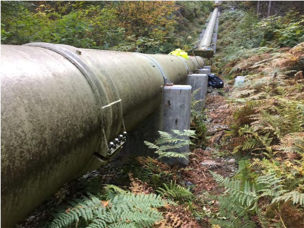
Photograph 6. Saddles 17 to 20; view to south toward Thrust Block III.
