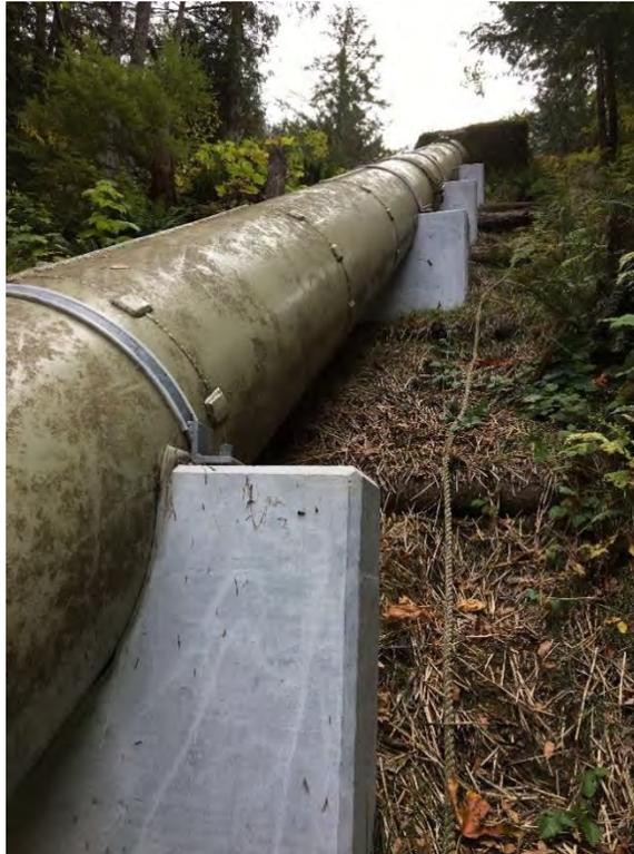
Photograph 2. Thrust Block II at top of hill, and Saddles 3 to 6; view to south.
