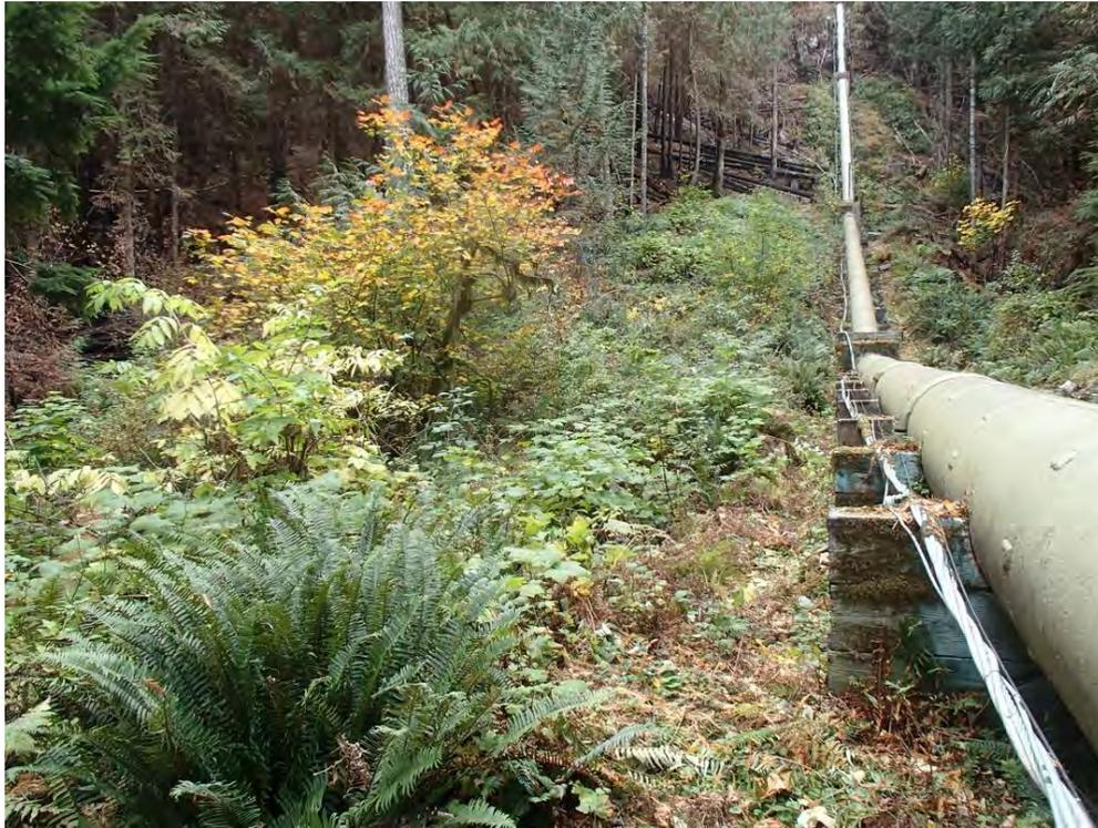
Photograph 3. Before saddle replacement: former creosote-treated wood saddles between Thrust Block II and III; view to south; October 2015.
