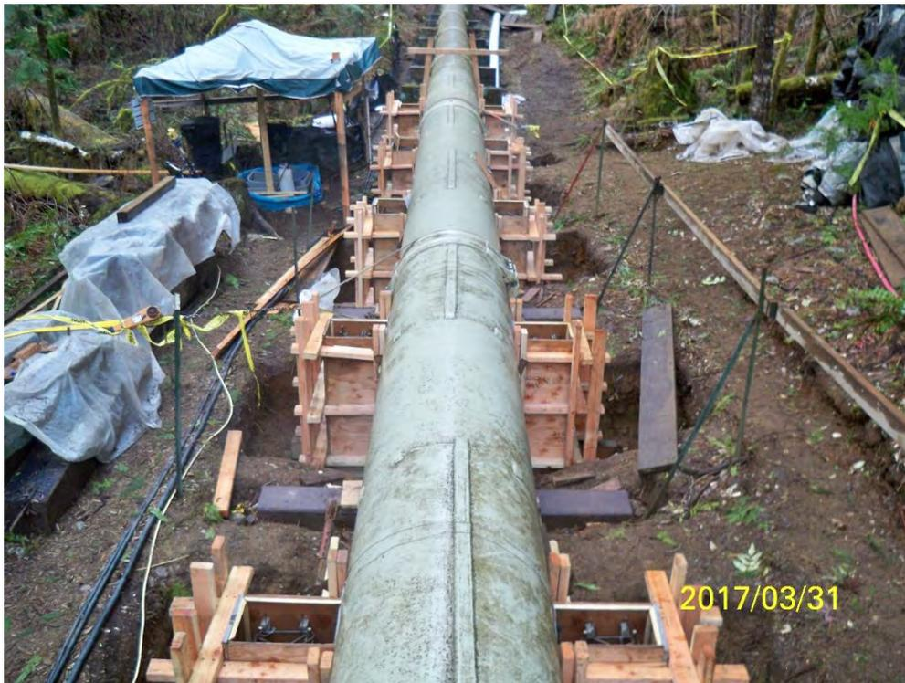
Photograph 4. During saddle replacement: soil excavation during saddle replacement; view to the south; March 2017.
