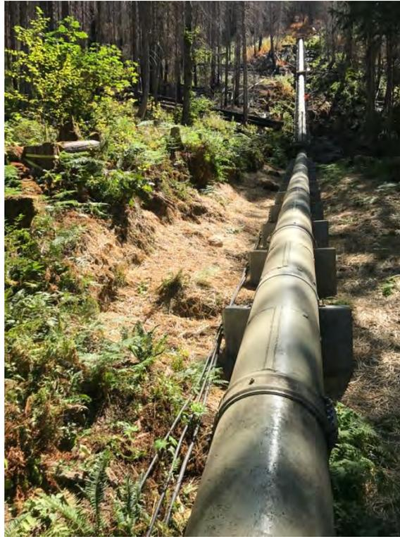
Photograph 5. After saddle replacement: between Thrust Block II and III just after saddle replacement; view to south toward Thrust Block III; September 2017.
